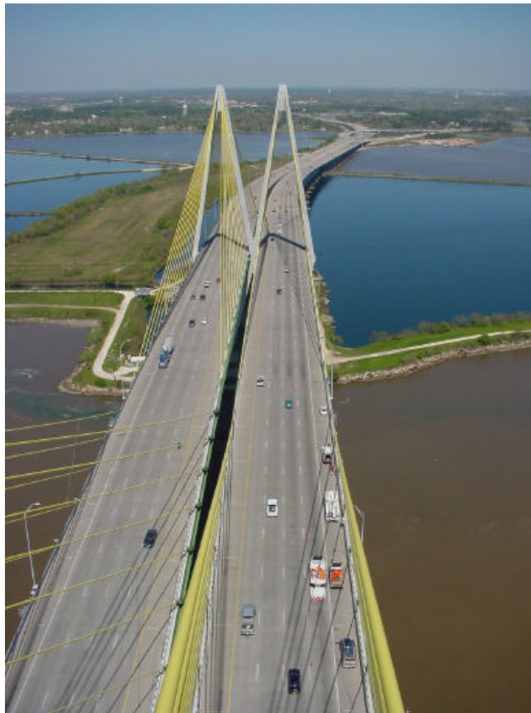
Figure 1.2 Two Independent Deck of the Fred Hartman Bridge
